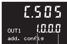
Additional configuration Out1:
